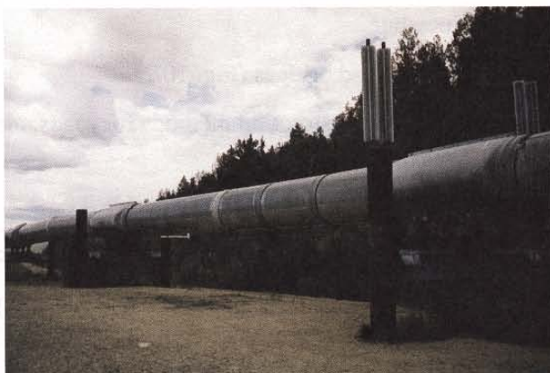
Figure 10.3. Trans-Alaska pipeline showing the above ground portion of the pipe supported by naturally refrigerated pilings. This expensive construction mode was required because of the presence of ice-rich permafrost which had to be kept frozen.
