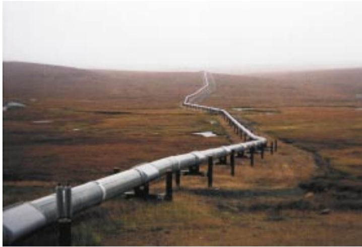
Figure 5. A section of the Trans Alaska Pipeline supported by vertical support members with thermosyphons in the ground. Note the fins on top of the support member whose function is to release heat transported up from the permafrost soil.
